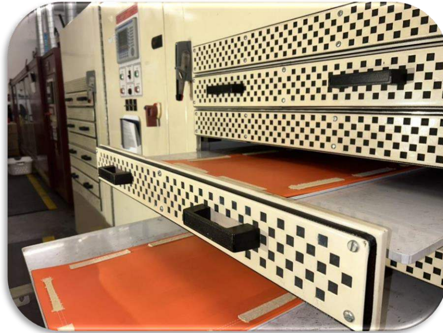
Figure 3 - Dielectric Testing of Blankets
